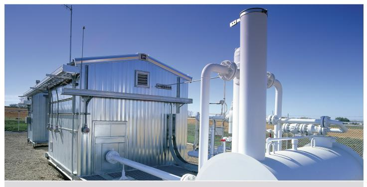
Meter stations are used to measure the volume and composition of natural gas transported through a pipeline.
